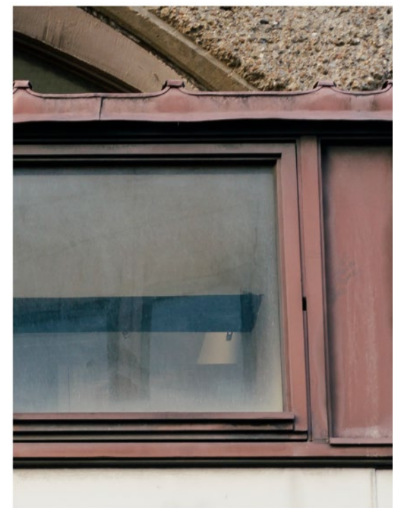
Original Window – no obvious rot
