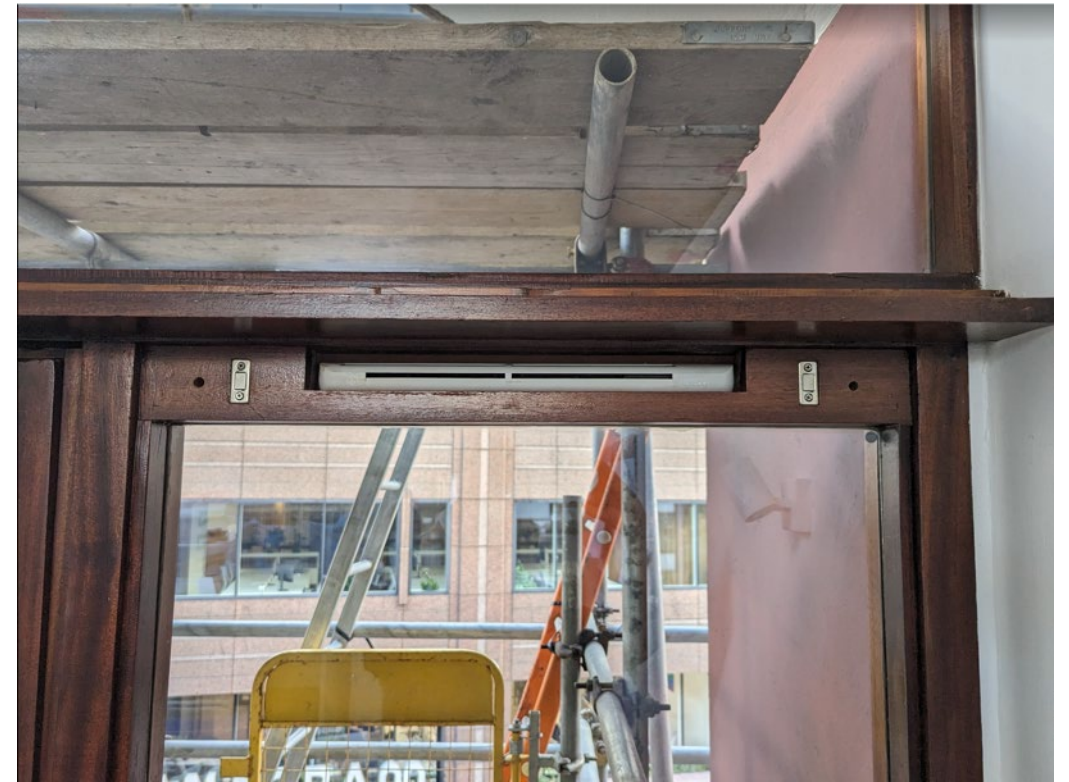
Trickle vent with sapele cover removed
