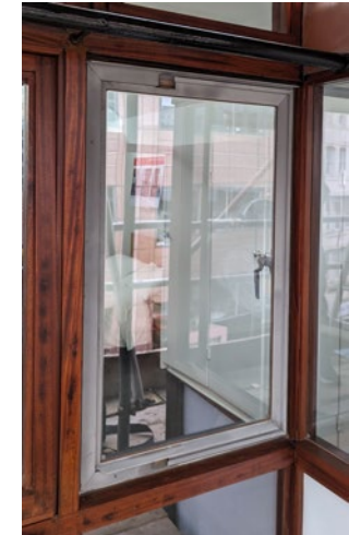
Existing window with VIG installed
